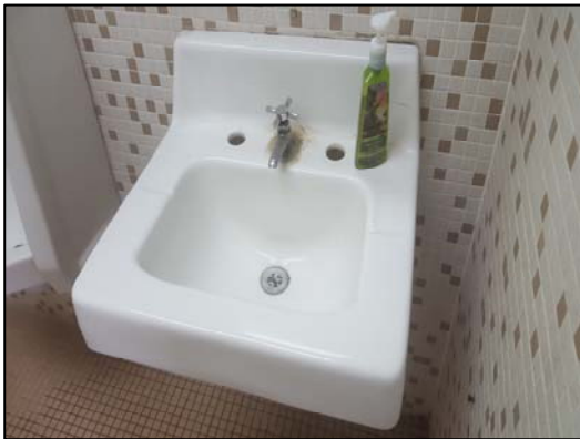
Medical Assistance Public Men's Bathroom Lead containing ceramic lavatory
