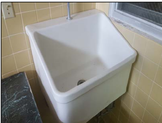
Newborns Delivery Room Area 1-23 Lead containing ceramic sink
