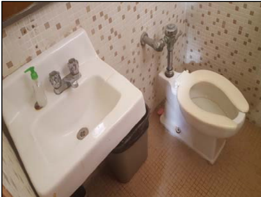
Medical Assistance Staff Men's Bathroom Lead containing ceramic lavatory & toilet
