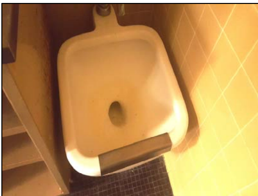
Newborns Delivery Room Area 1-5 Lead containing ceramic sink
