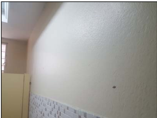
Medical Assistance Public Women's Bathroom Lead based painted concrete wall
