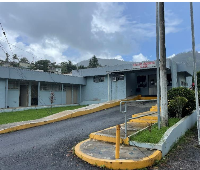
Yellow Concrete Curb, Riser and Bollard Painted with LBP Emergency Area, Exterior
