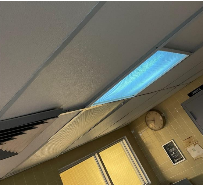
Typical Asbestos Containing Ceiling Tiles 2'x 4' (Transite)
