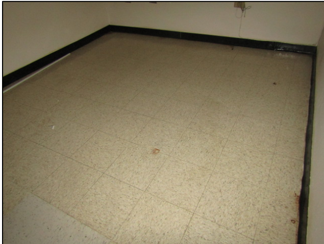
Delivery Room Areas Asbestos-containing cream vinyl tiles (12x12) & associated mastic.
